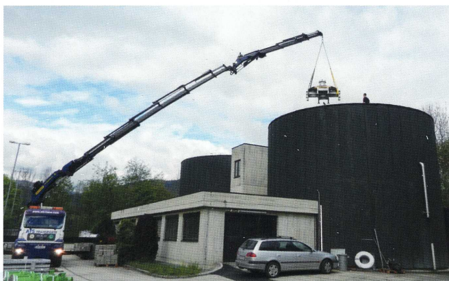
Montage Gashaube Faultürme
