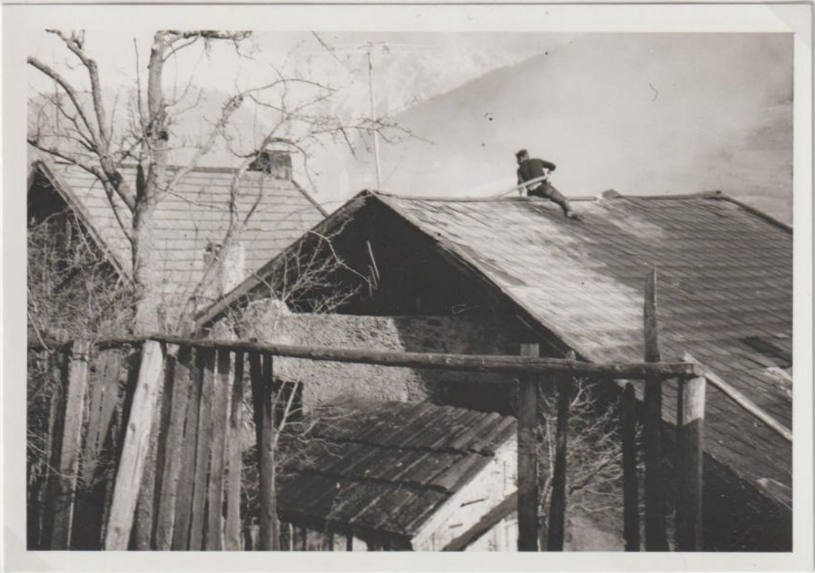
A view from the roof of the old building (Hill)
