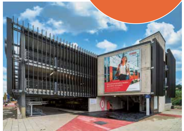
Neues Parkhaus in Jenbach. © ÖBB - Sailerbrothers.
